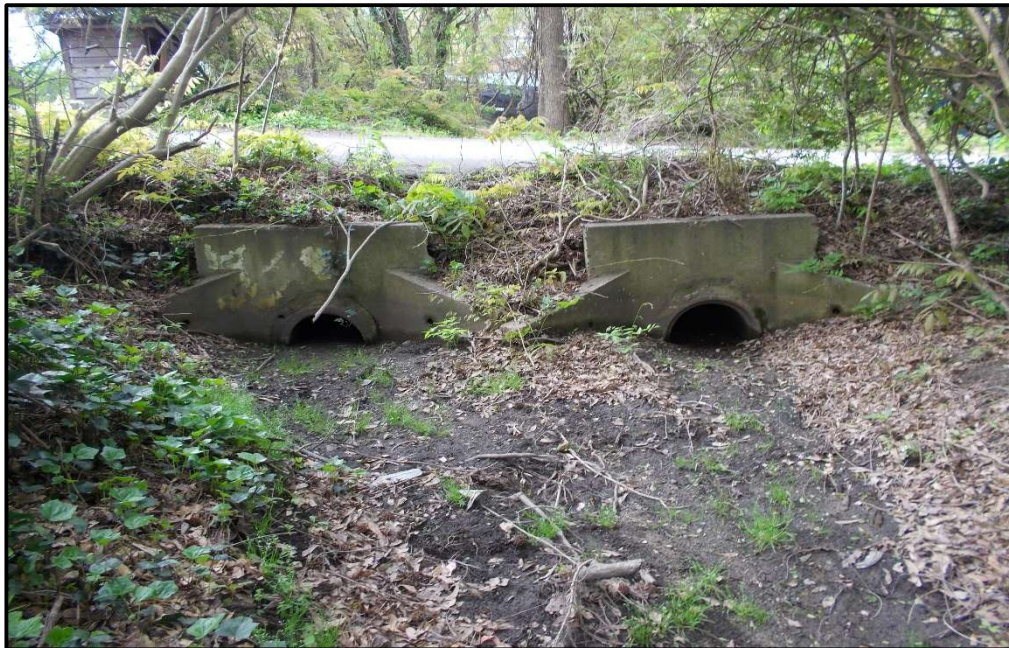
Photograph 002. Two 18-inch culverts at non-buffered state water (facing south). (4/21/22)
