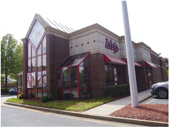
BUILDING TO THE NORTH
