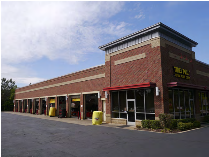
BUILDING TO THE NORTH
