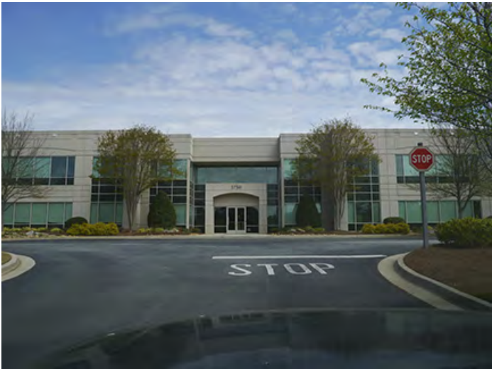
BUILDING TO THE WEST
