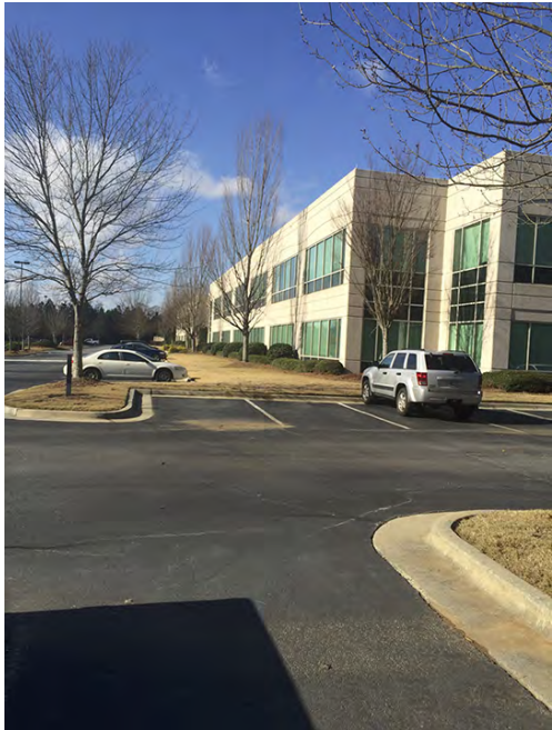
BUILDING TO THE WEST
