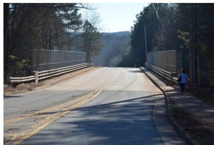
Figure 11. Encore Parkway Bridge before renovation provided a narrow sidewalk abutting the travel lanes
