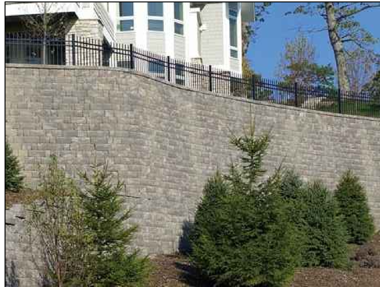
MODULAR BLOCK RETAINING WALL - ANCHOR DIAMOND PRO
