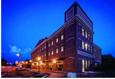
Figure 6. Milton Avenue Parking Deck (275 spaces), police substation, and retail condominium spaces fronting onto Milton Ave.
