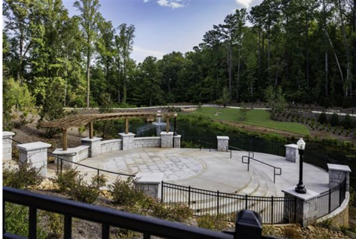
Figure 8. Photo of Thompson Street Park. The park sits in the center of the 1-mile trail connection from Downtown to Avalon and was constructed by a private developer in exchange for development impact fee credits. The pond serves as a detention pond.
