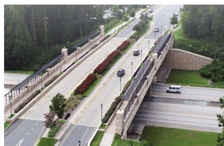
Figure 12. The Encore Parkway Bridge now has a single travel lane in each direction, provides an in-street bicycle lane and added a landscaped planter separating the travel lane from the widened sidewalk.
