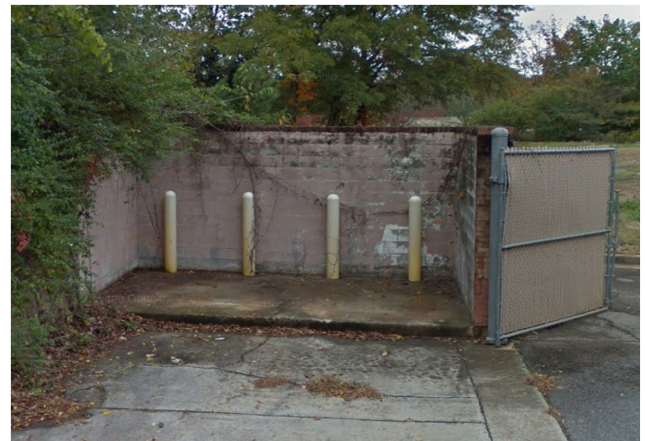
EXISTING DUMPSTER ENCLOSURE CONDITIONS
