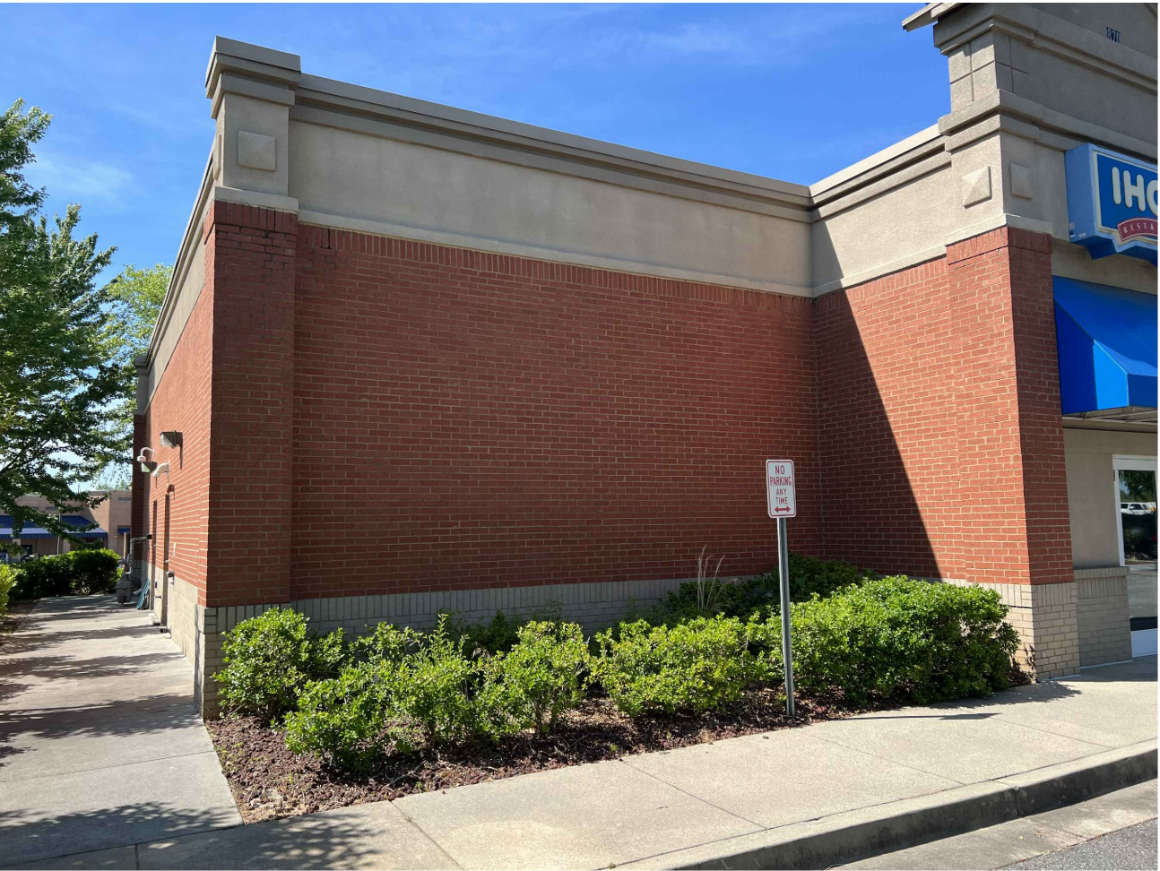
06 - EXISTING SOUTH CORNER
