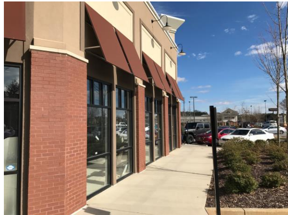
4. Existing sidewalk | No alteration
