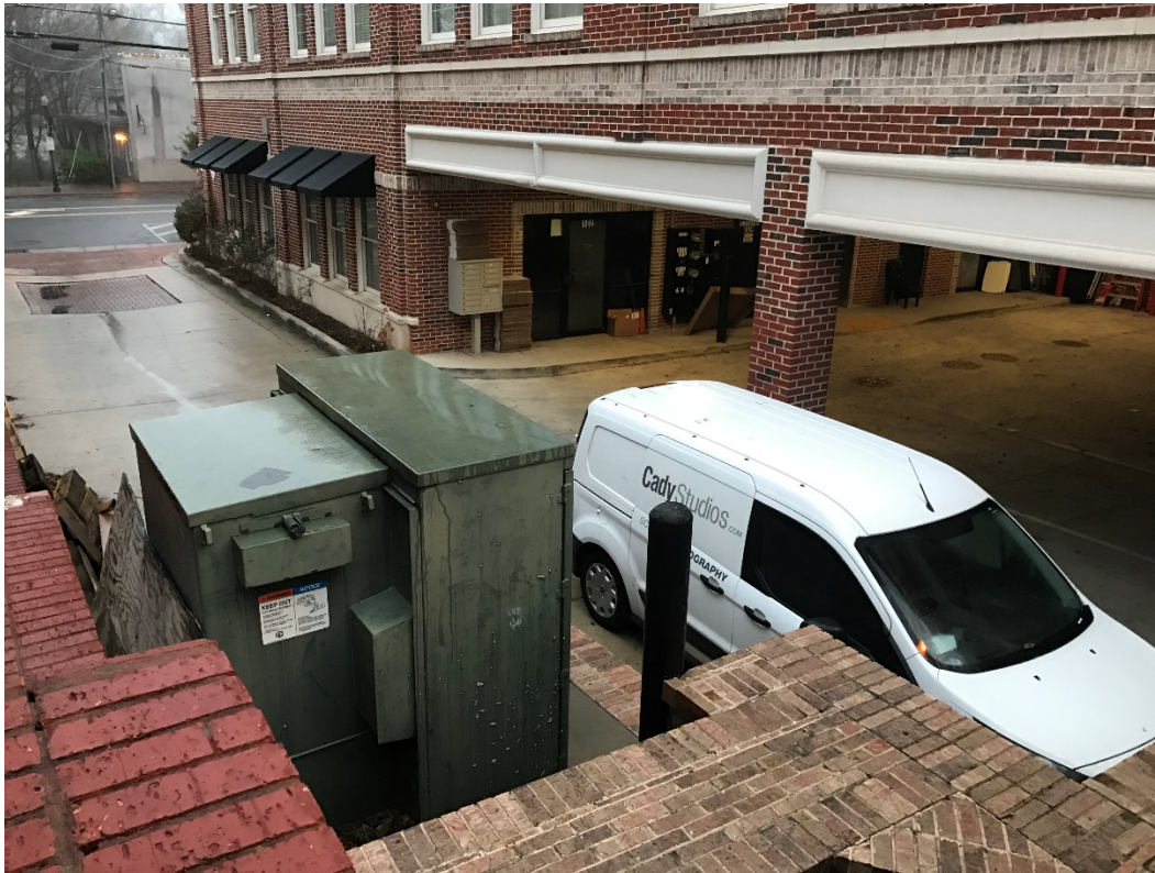
3. Existing Alley Overview | Parking Entry | Infill Area
