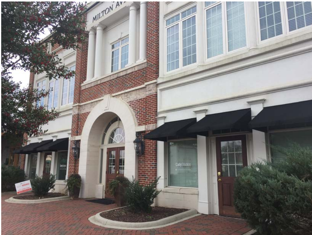
1. Existing Front Façade
