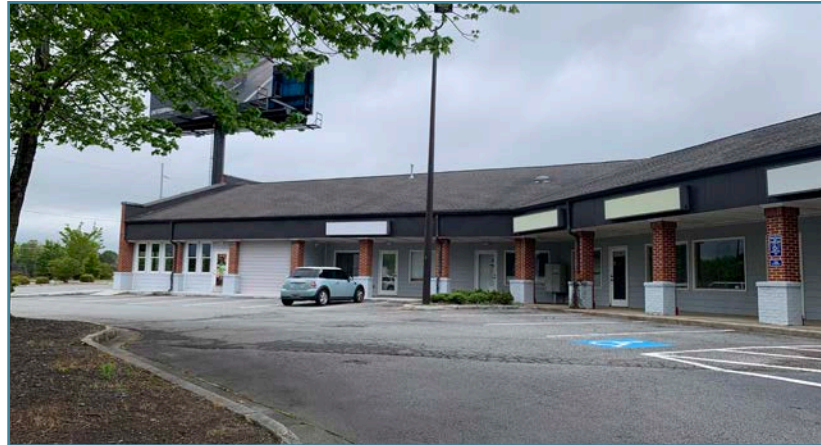
Shopping Center along South Main Street
