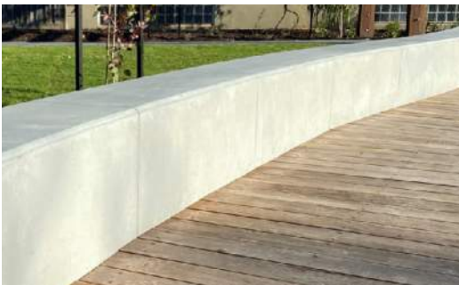
W2 Concrete Seat Walls
