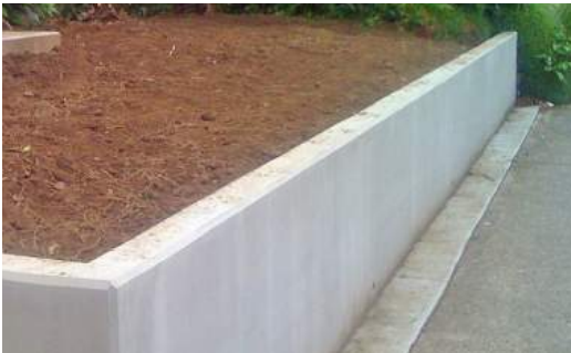
W1 Concrete Retaining Wall
