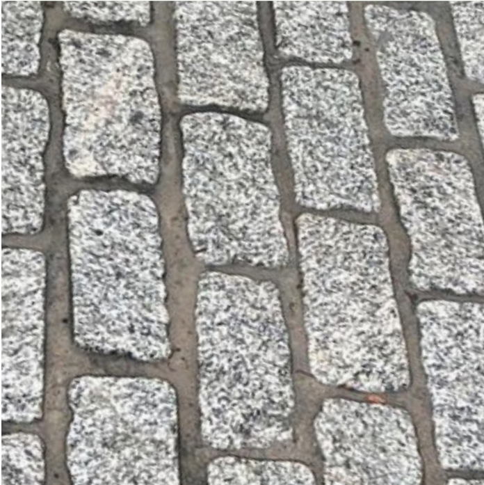
GRANITE BLOCK SETTS • Old Roswell Shared Street Runnel • Street Tree Pits • Buffer Strips (< 2FT Width)
