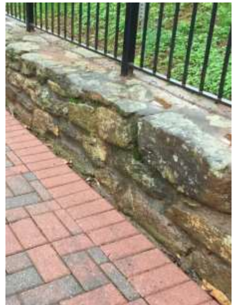
Cut stone cap detail & seat wall
