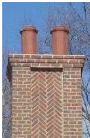
Brick chimney & chimney pot detail.
