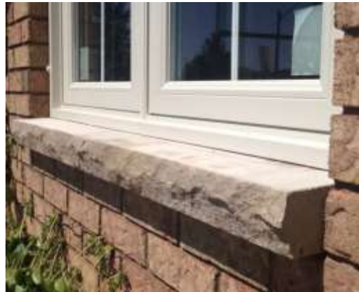
Cut stone window sill detail
