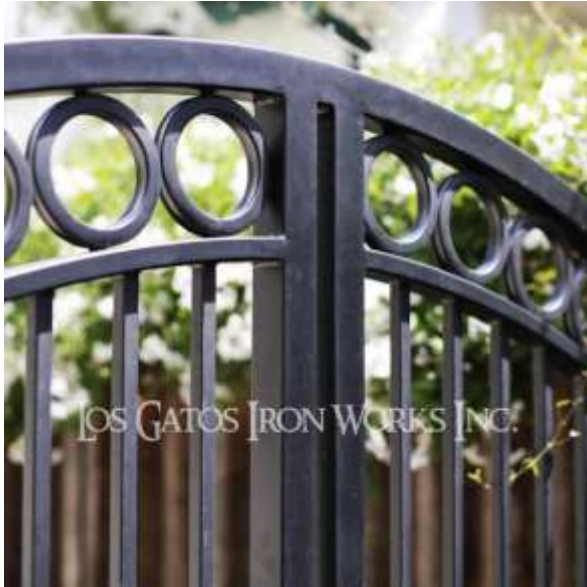
Typical exterior porch rails & gates:
