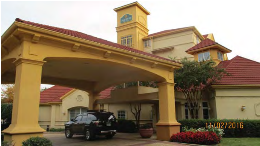
EXISTING PORTE COCHERE ELEVATION
