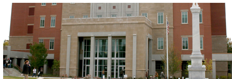
CARROLL COUNTY COURTHOUSE RENOVATION $3M; 26,000 SF
