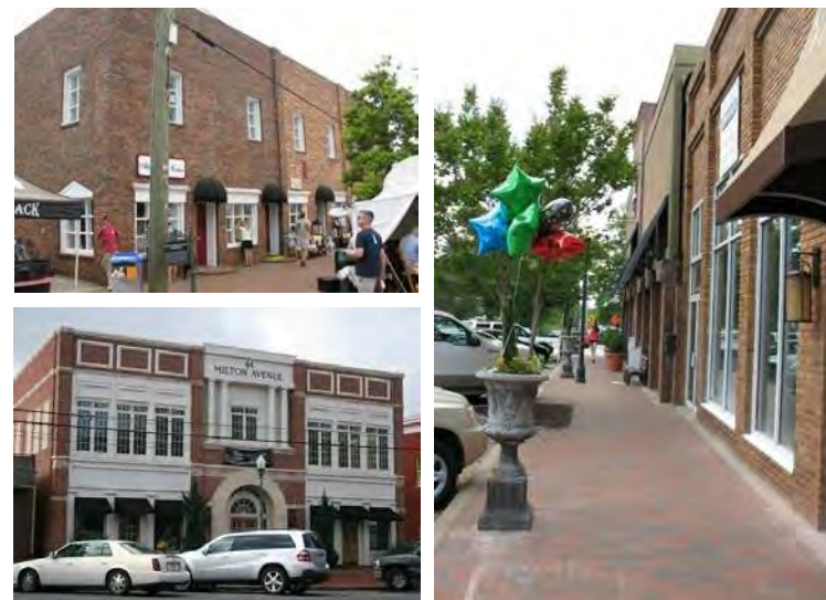
Buildings and streetscape within Alpharetta's existing downtown.
