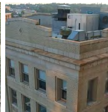
A detailed wall, setback from the sidewalk, screens a loading area and encloses a landscaped seating zone (Right). Rooftop equipment is set back from the parapet to screen its visibility from the public street (Left).
