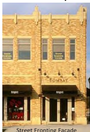
Street Fronting Facade
