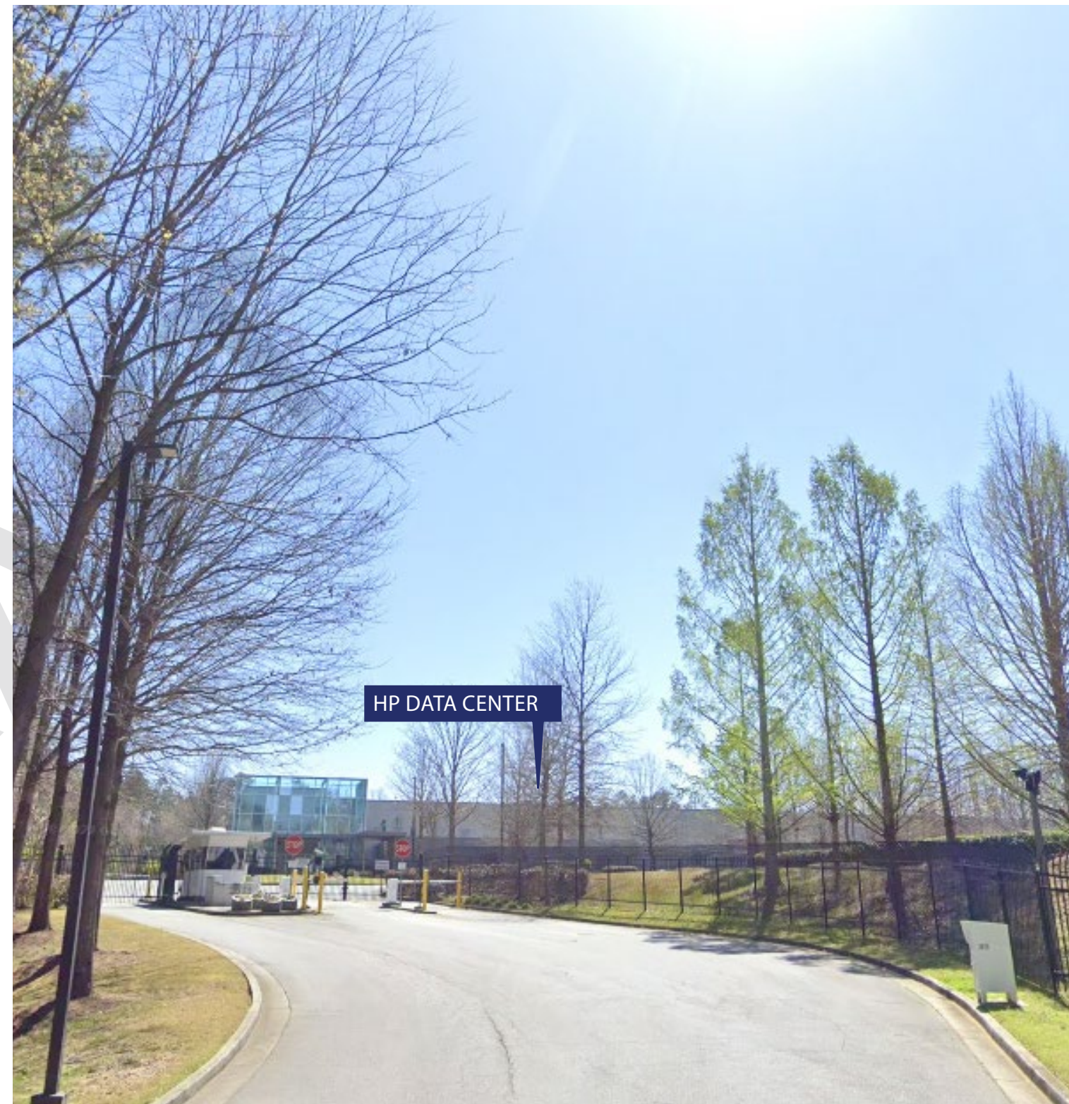
SOUTH - TOWARD HP DATA CENTER
