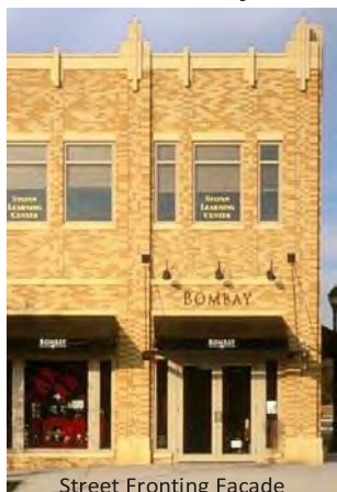
Street Fronting Facade
