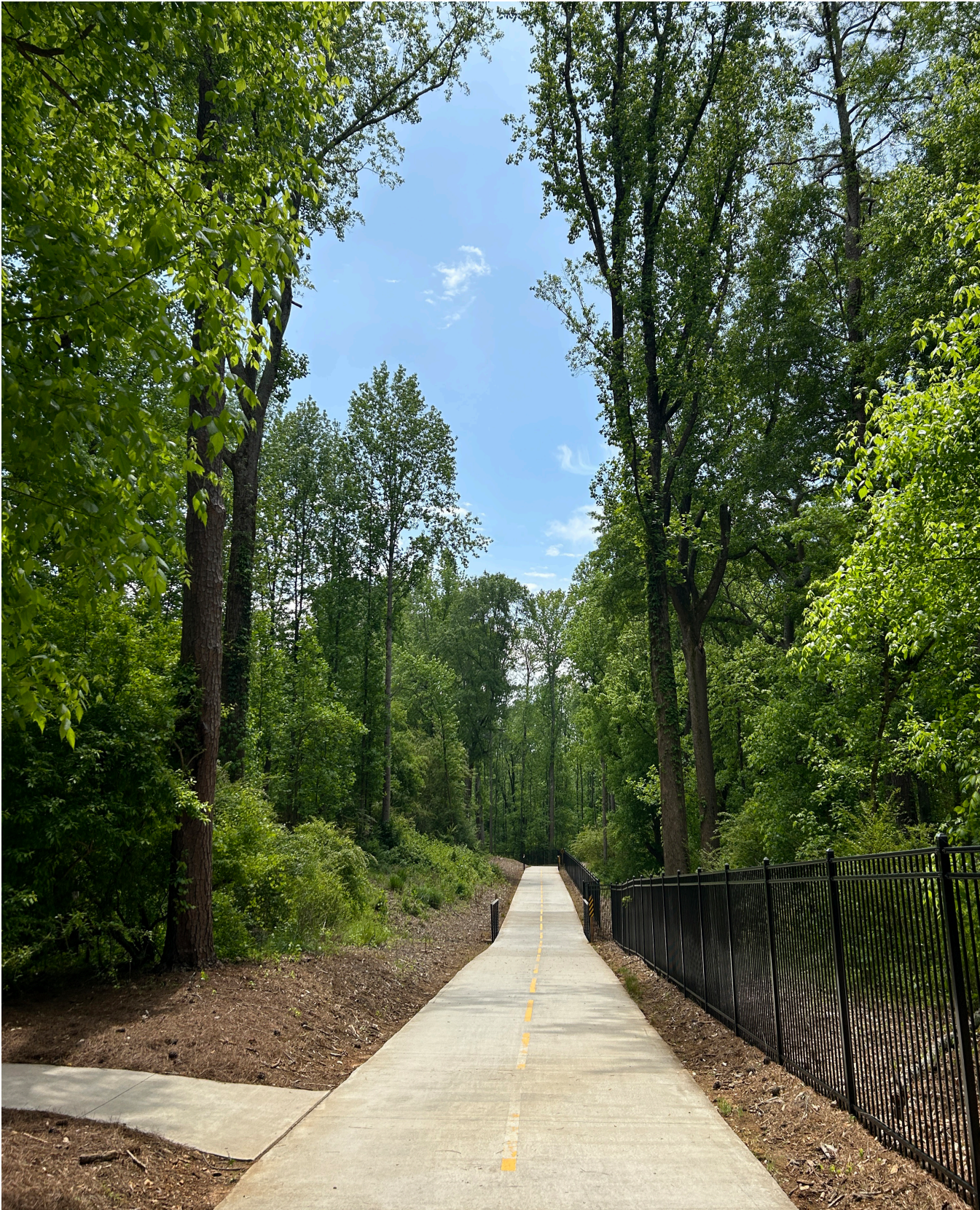
The Big Creek Greenway lines the southern edge of the Windward Tech District and has become an important local amenity.
