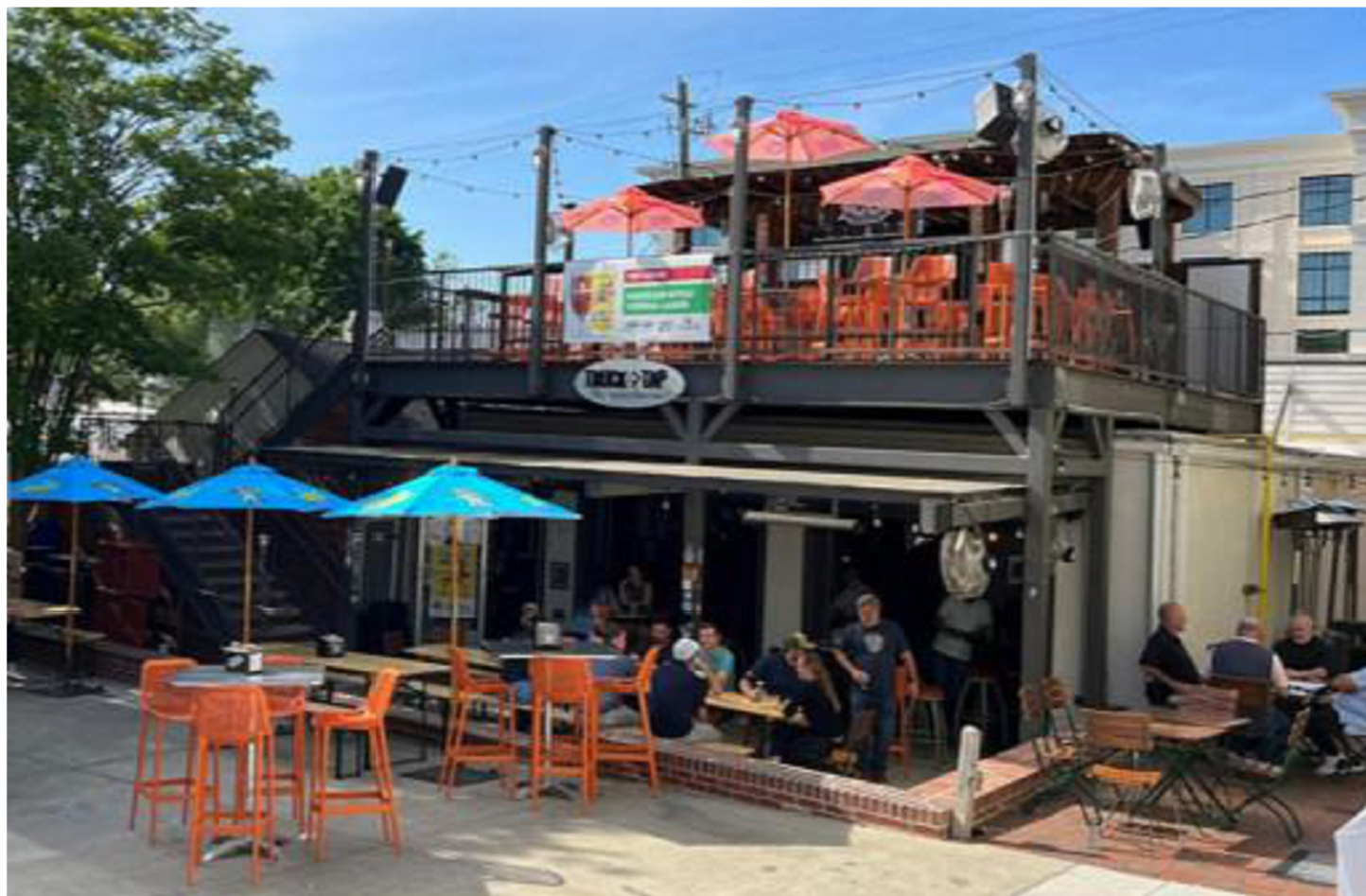
EXISTING ROOF TOP PATIO
