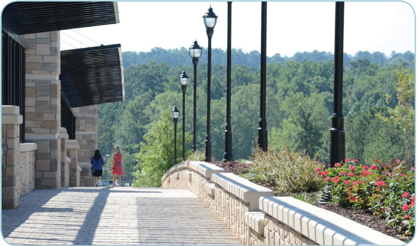
Encore Parkway Bridge, completed 2017
