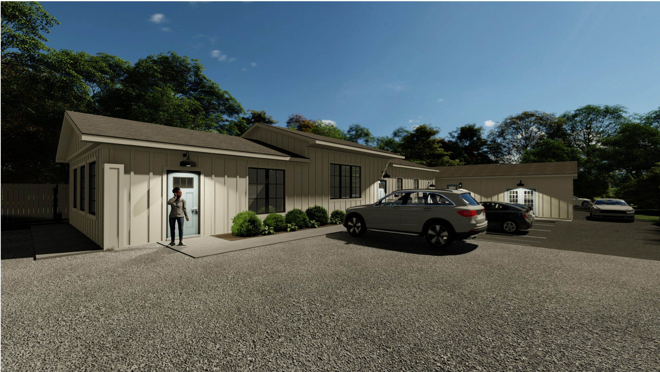
Facade W | View from Parking Area
