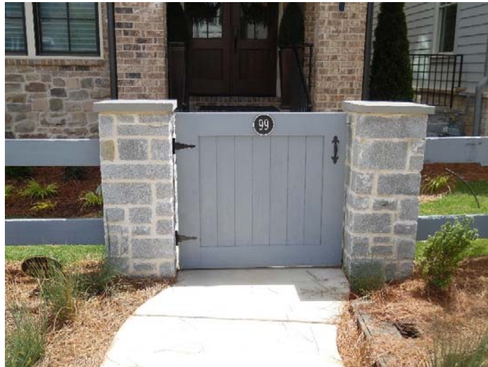
On Site Example of Granite Column with Bluestone Cap
