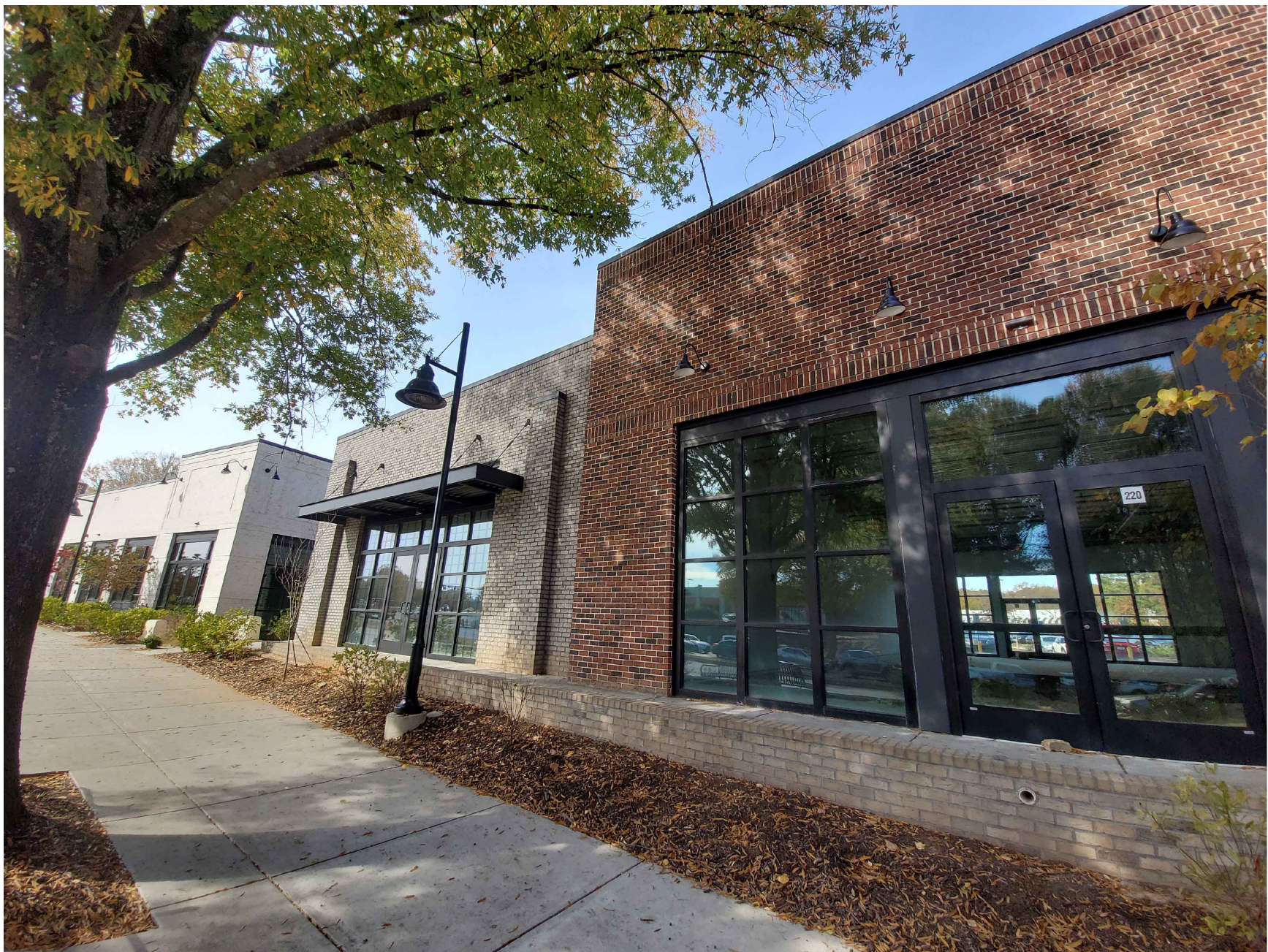
VIEW TOWARDS EXISTING EXTERIOR SOUTH FACADE
