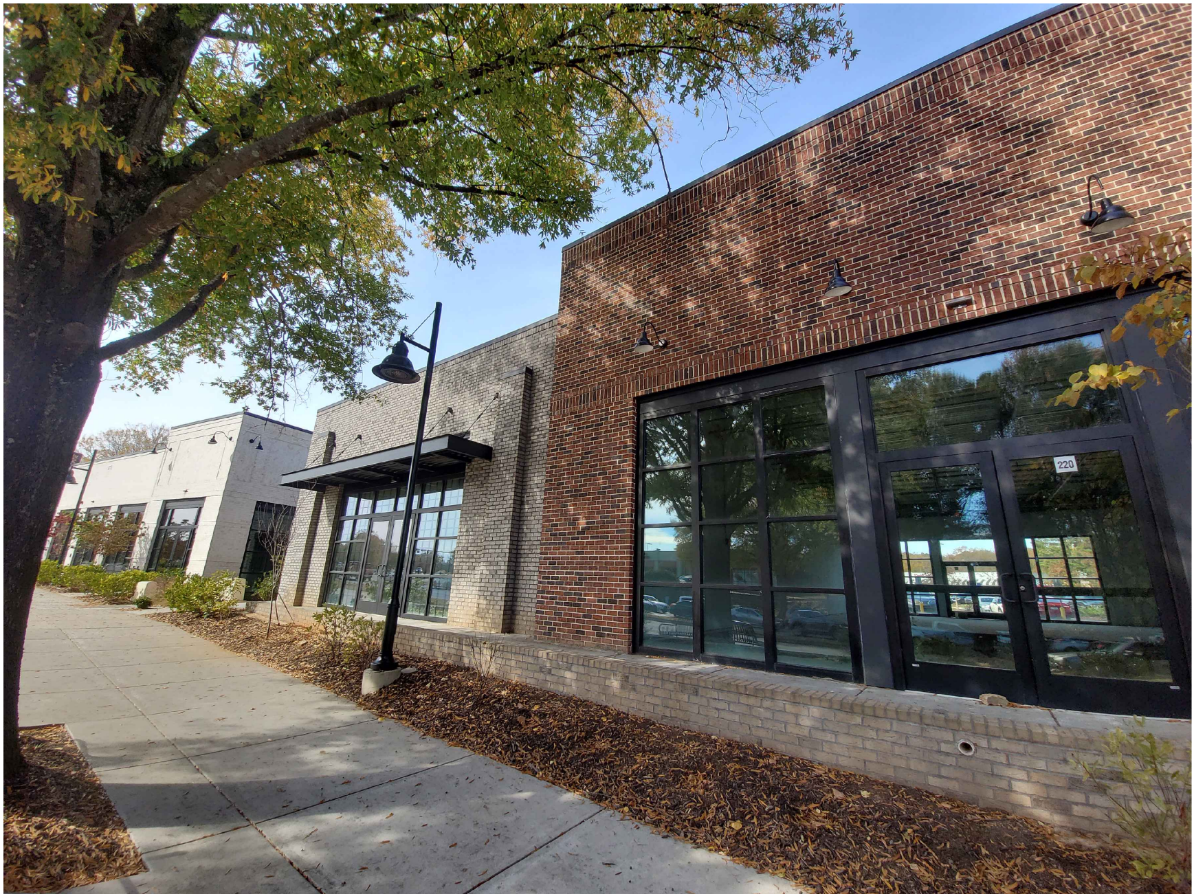
VIEW TOWARDS EXISTING EXTERIOR SOUTH FACADE
