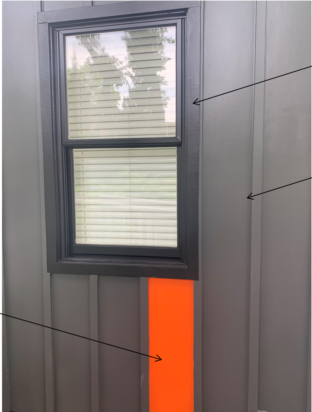
ACTUAL PAINT MOCK-UP ON BACKSIDE OF BUILDING
