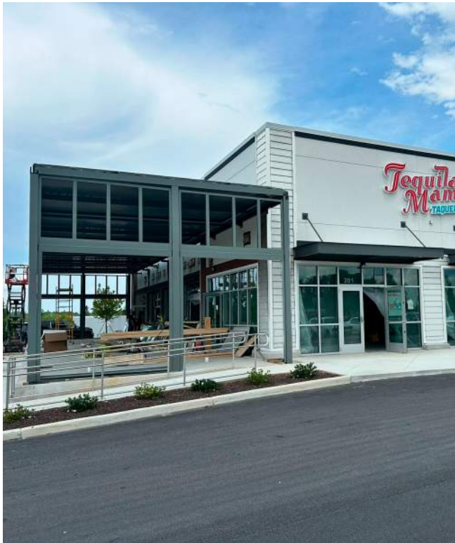
GUILLOTINE WINDOW SYSTEM - EXISTING LOCATION
