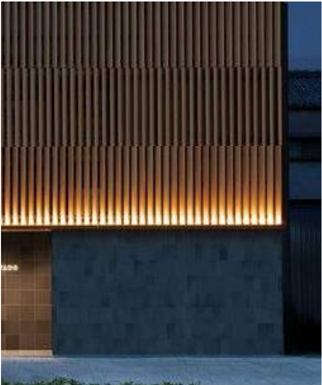
EXTERIOR LIGHTING - UPLIGHTS + SPOT LIGHT
