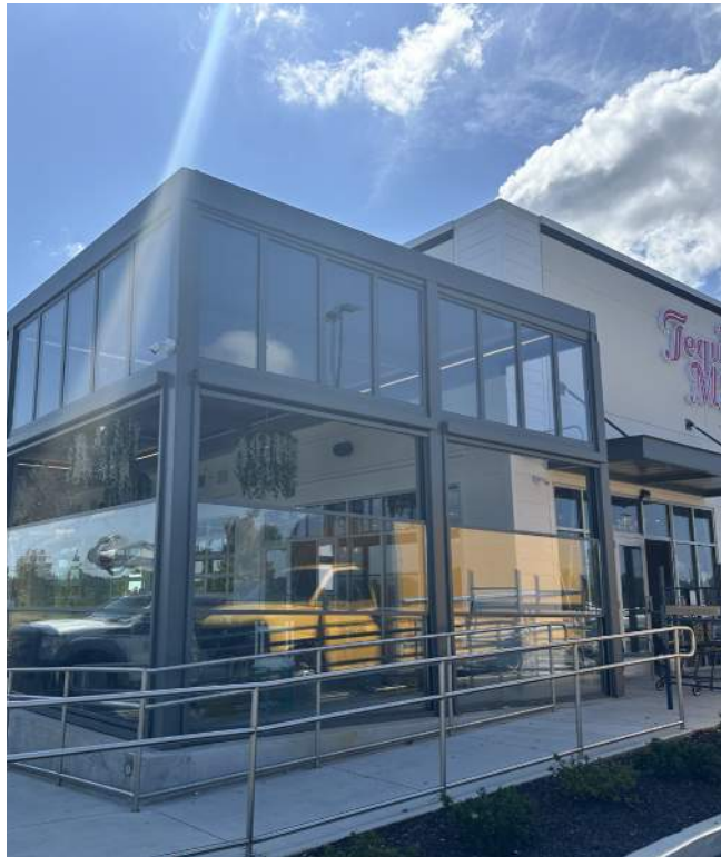
GUILLOTINE WINDOW SYSTEM - EXISTING LOCATION
