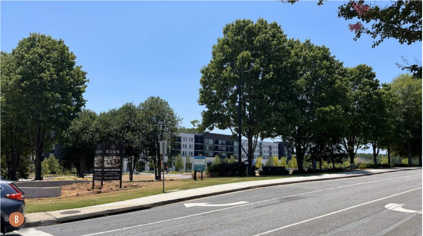
VIEW FROM LAKEVIEW PARKWAY AND HAYNES BRIDGE RD INTERSECTION
